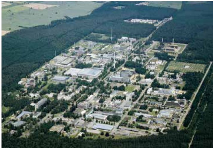
View of the Research Center Karlsruhe (Campus North)
